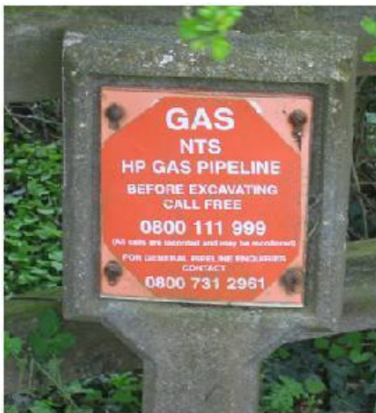
Marker and aerial marker Post signifying the presence of underground services, found on boundary lines
