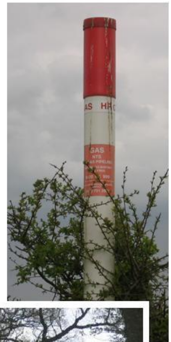
Marker and aerial marker Post signifying the presence of underground services, found on boundary lines
